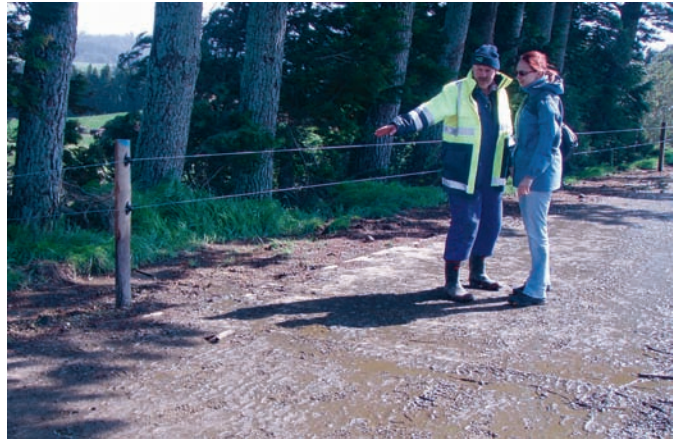
Lachlan McKenzie pointing out a smooth transition line (pumice race to concrete) and pothole free race surface after close to 2m of rain in the past three months.
